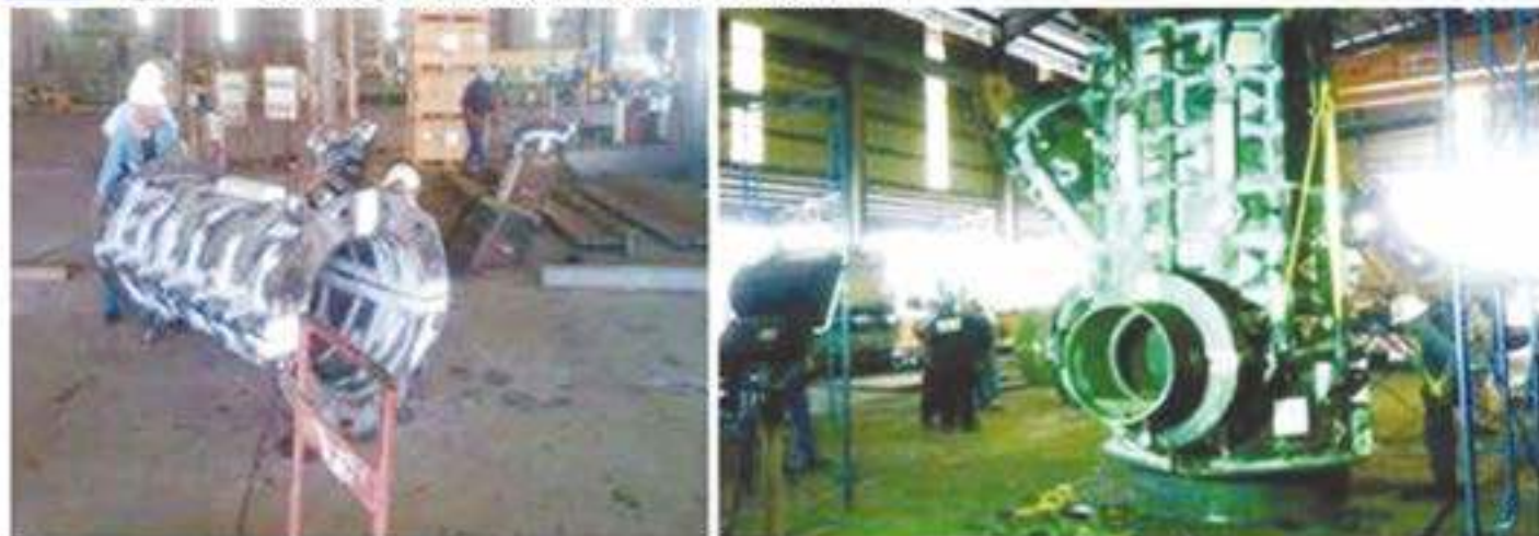
02 GUMUSUT KAKAP: FABRICATION AND INSTALLATION OF 72 UNITS SKID BEAM
