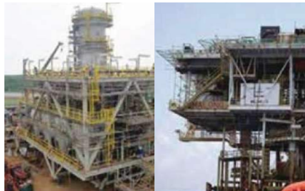
FABRICATION AND INSTALLATION OF STEEL STRUCTURE, PIPING AND EQUIPMENT
