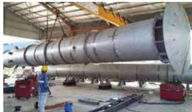
FABRICATION OF GTG & GTC EXHAUST DUCT FOR FPSO CHENDOR TOPSIDE
