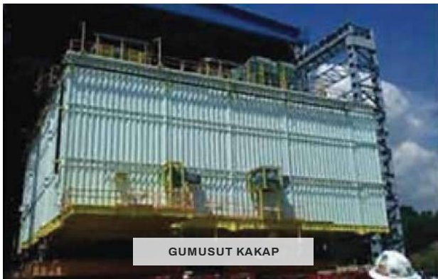
FABRICATION OF PERMANENT LIVING QUARTERS, PIPE SUPPORT, GRILLAGE
