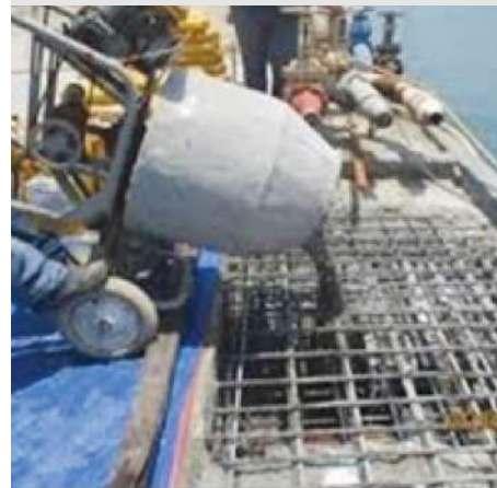
PILE JACKETING & JETTY BERTH 6 & 7 KEMAMAN SUPRA PORT GALIAN S
