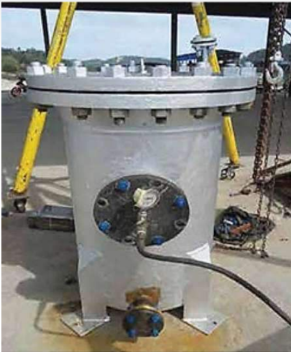
REPAIR OF STRAINER HOUSING STR-1201 FOR VCMSB
