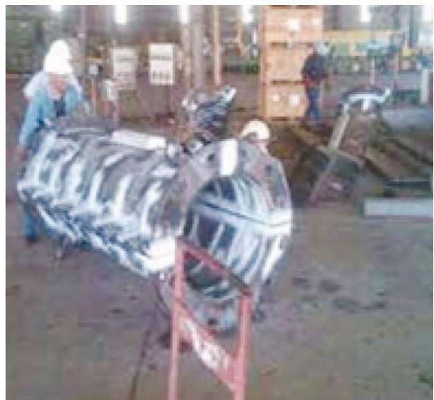
01 MODIFICATION WORKS OF NODE CLAMP FOR BRA CCP JACKET NODE / TALISMAN
