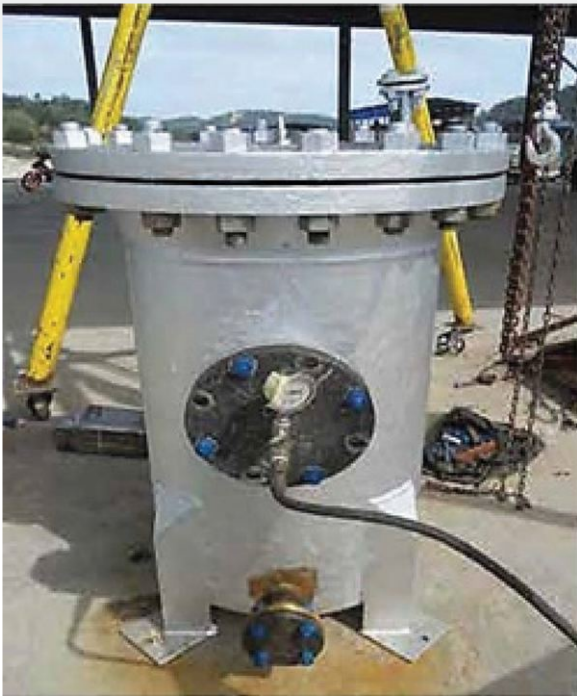
REPAIR OF STRAINER HOUSING STR-1201 FOR VCMSB
